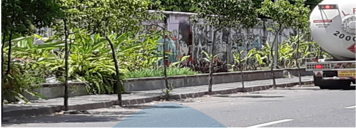
Figure 2.2.1 Pavement on Jalan Raya Utama
