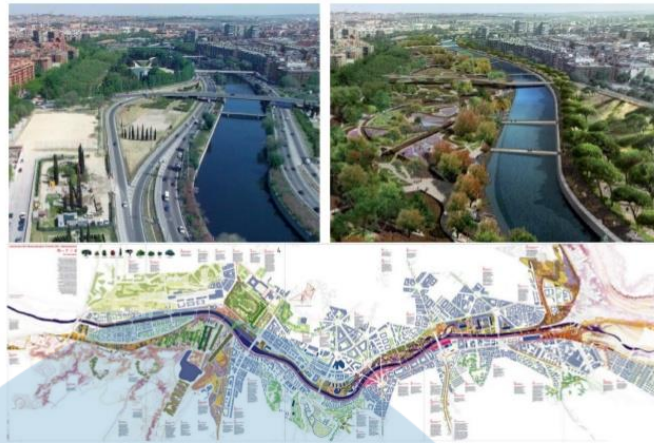
Motorways. Under: M30 ...and over Madrid Rio Landscape 2007-2011 (B&G, R&AS, West 8)
