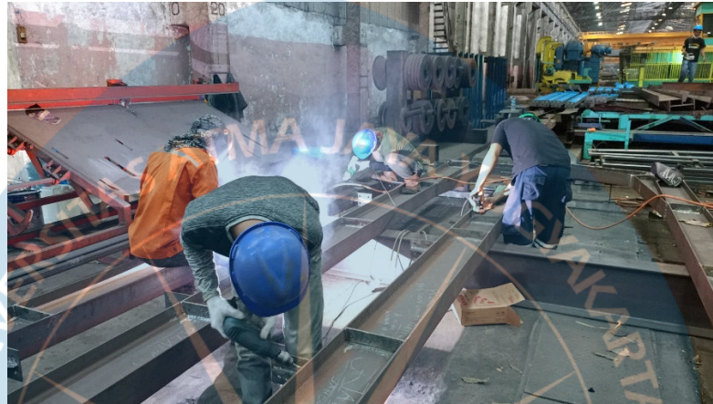
Figure 2.9 Welding Repair Inspection of Warehouse Fabrication
