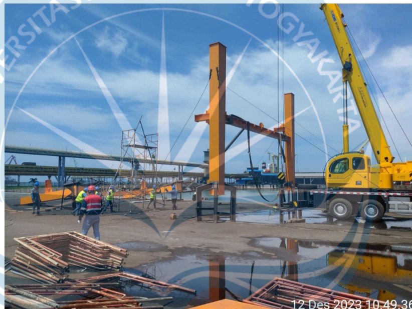
Figure 2.17 Coal Hopper Erecting
