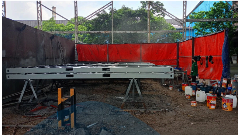
Figure 2.12 Sandblast and Coating Checklist of Wika Modular
