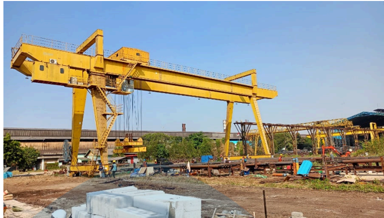
Figure 2.30 20-Tons Load Capacity Girder Crane
