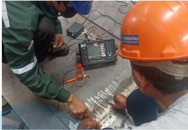
Figure 2.19 Ultrasonic Examination Girder Plate
