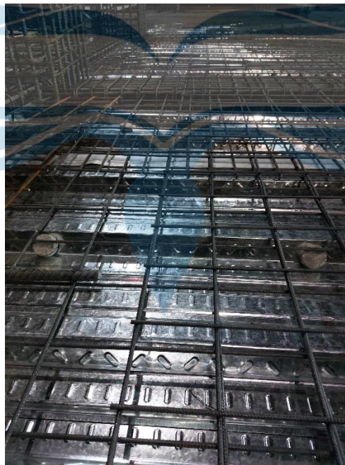
Gambar 2. 27 Besi Dowel, Cakar Ayam, dan Beton Decking
