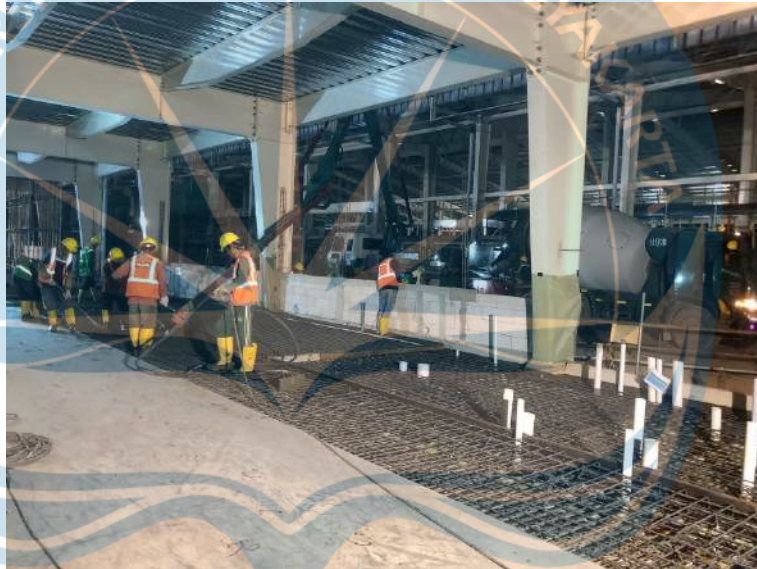
Gambar II. 22 Monitoring Pengecoran Beton
