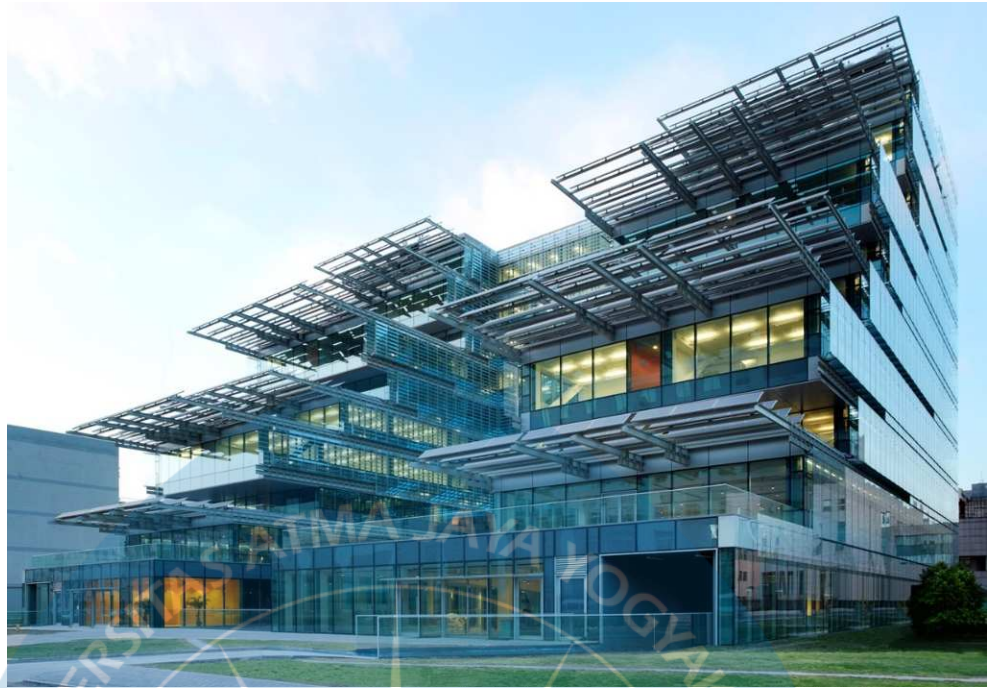
GAMBAR 3. 5 Sino-Italian Ecological and Energy Efficient Building
