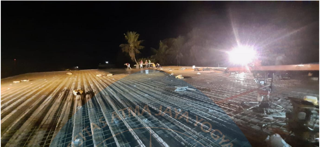
Figure 2.6.3 Preparations for the third-floor concrete
