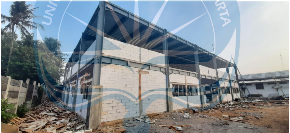
Figure 2.6.13 Condition outside building after the wall polish
