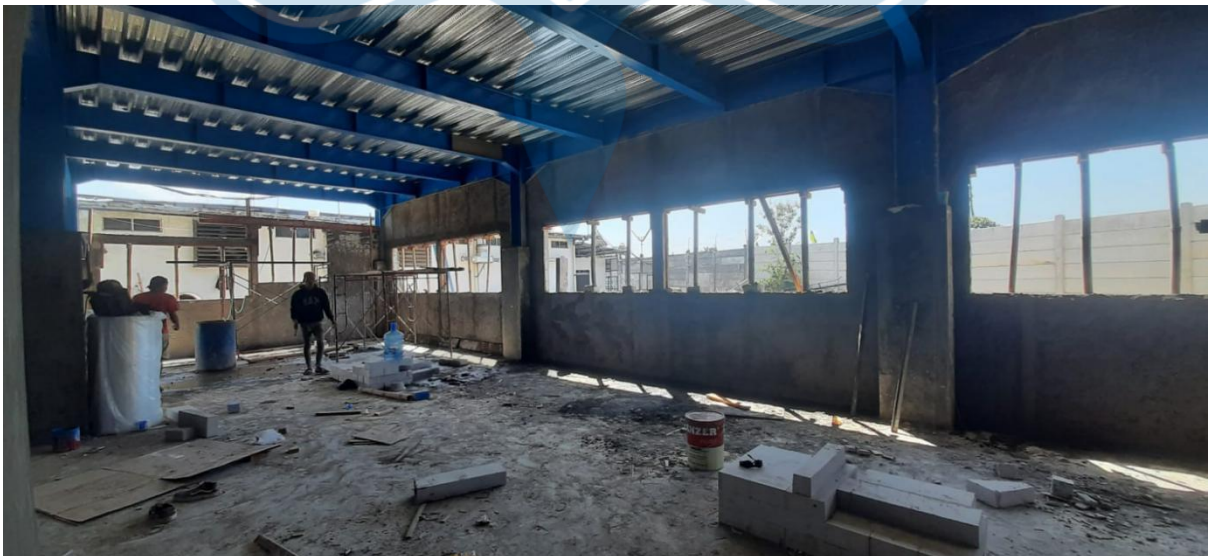
Figure 2.6.11 Polishing the wall on the first floor (1 week work)
