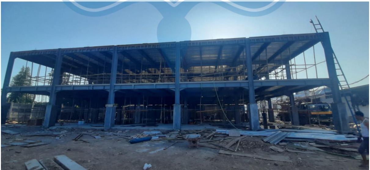
Figure 2.6.2 Site Project Conditions without any walls just steel structure.
