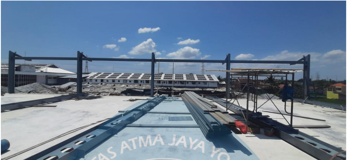
Figure 2.6.14 Third floor condition before the roof installation
