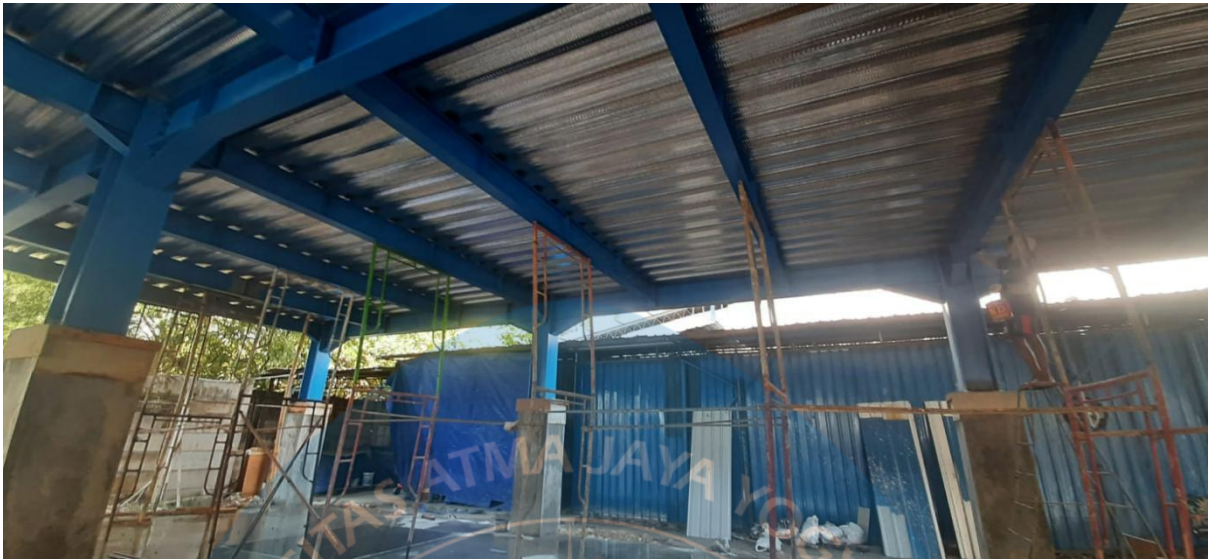
Painting the column and beam to avoiding the rusting
