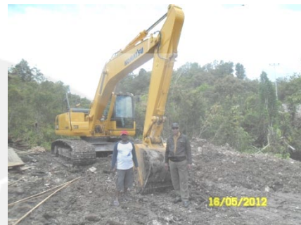
Galian Saluran Drainase
