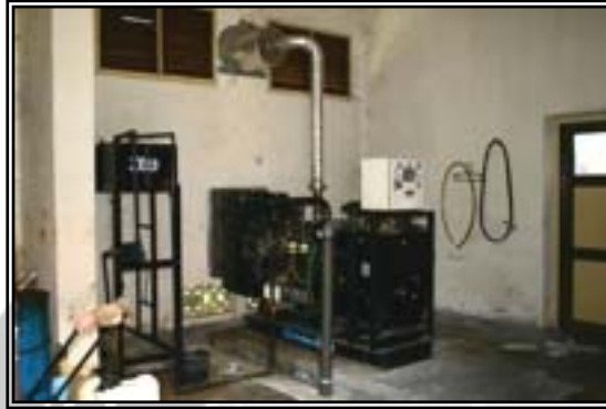
Gambar : 2.57 Ruang Genset Sumber : http://www.pantisemedi.com
