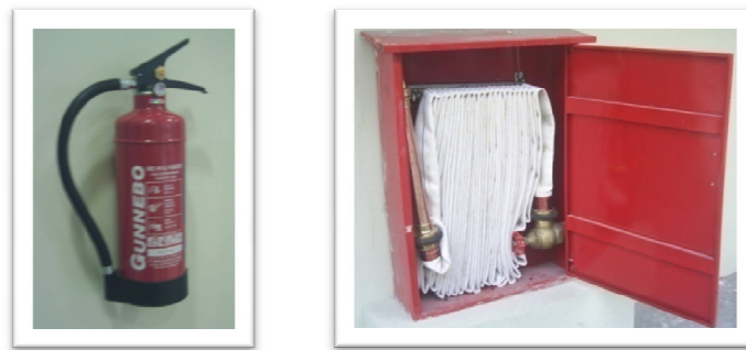
Gambar: 5.20 Portable Fire Extinguisher, dan Hydrant box
