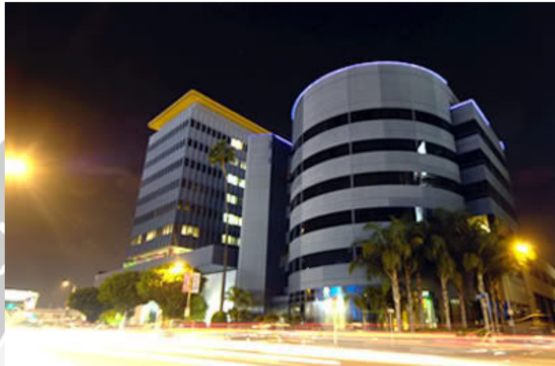
Gambar II.6 Gedung Los Angeles Film School.
