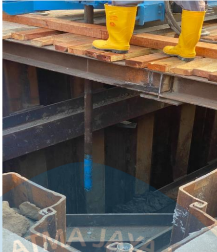
FIGURE 2.6 Jet Grouting
