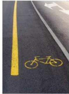
**PENGECATAN ASPAL DENGAN CAT REFLEKTIF DAN PEMBERIAN REFLEKTOR**
