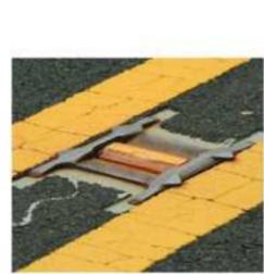
**PENGECATAN ASPAL DENGAN CAT REFLEKTIF DAN PEMBERIAN REFLEKTOR**
