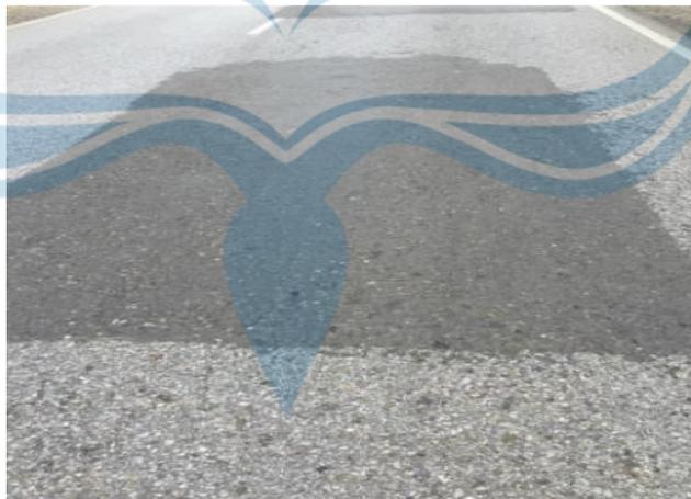
Gambar 2.13. Rusak Tambalan (*Patching end Utiliti Cut Patching*)
