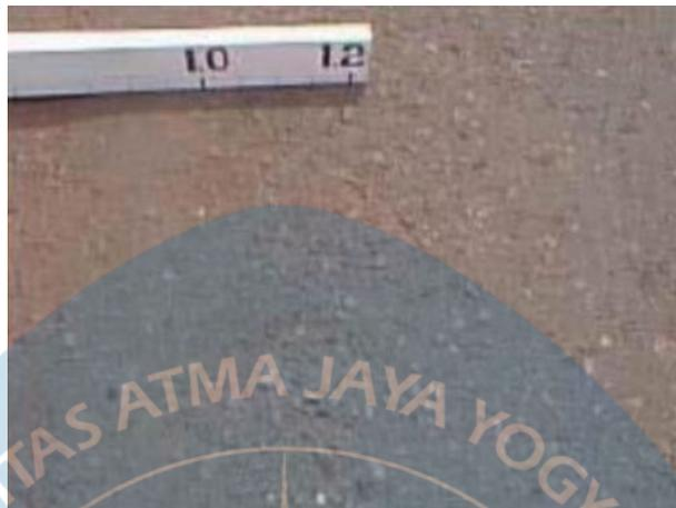
Gambar 2.14. Rusak Pengausan Agregat (*Polished Agregat*)
