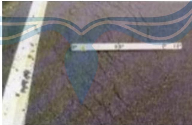
Gambar 2.19. Rusak Patah Slip (*Slippage Cracking*)
