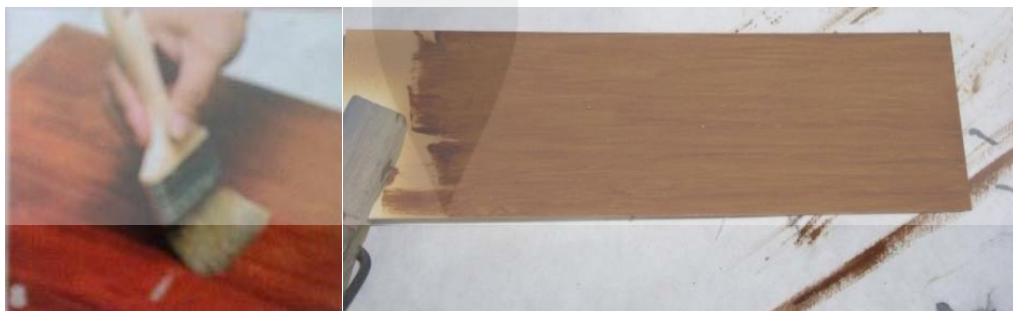
Gambar 2.6 Proses Base Coat
