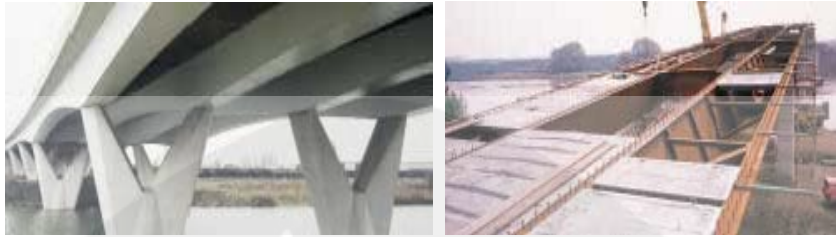
Gambar 2.5. Jembatan gelagar kotak ( box girder ), multi span.
