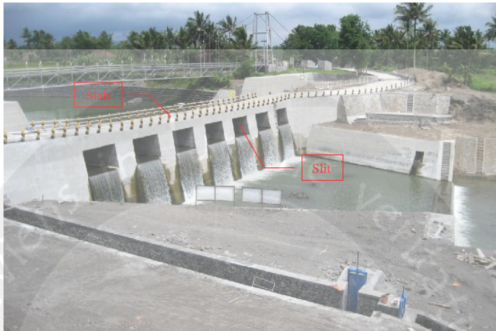
Gambar 1. Sabo dam PA-C Srowol
