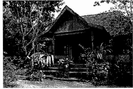
Figure 5-26 A house in Pakem that applies an elevated floor system by raising the ground level. Thus, unlike other traditional styles in Indonesia, Javanese buildings do not utilize the space under the floor.
