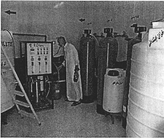
Fig 15 Small water-purification plant Building.
