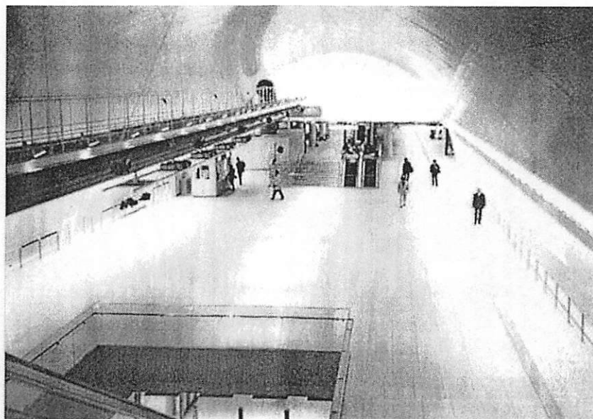
Fig2: Minatomirai Station on Minatomirai Line in Yokohama
