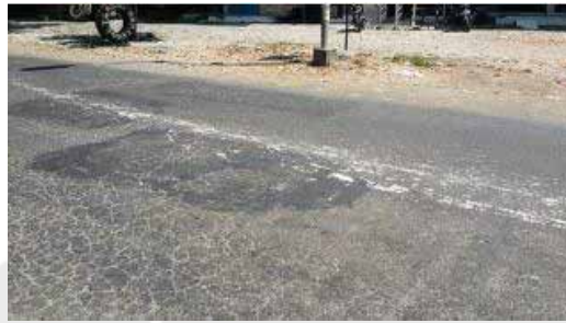
Gambar 2.4. Kerusakan Joint Reflection Cracking
