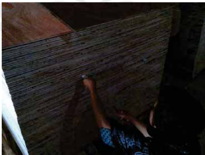
Gambar 9. Proses repair core void
