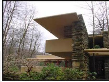
Gambar 4.2 Falling Water House KantileverCantilever
