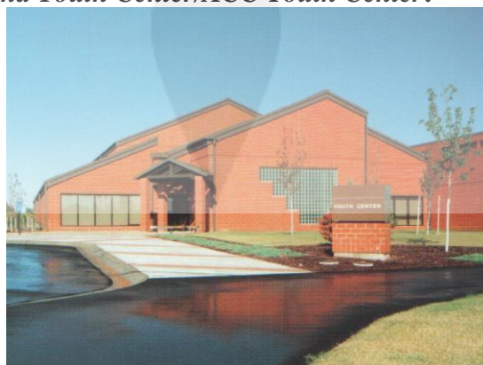
Gambar II.8. Tampak Air Combat Command Youth Center Sumber: (Air Combat Command, Directorate of Services)
