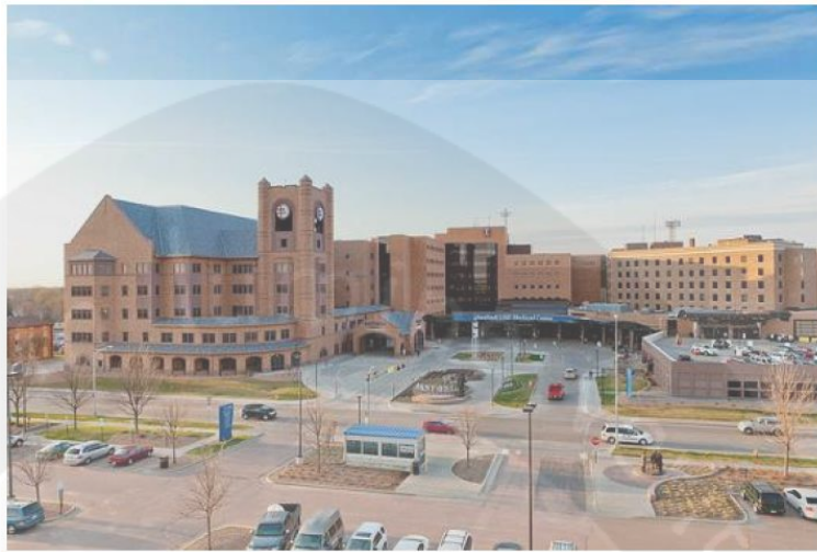
Gambar 2.1 : Eksterior Sanford Heart Hospital Sioux Falls (Sumber : http://www.flickr.com/photos/sanfordhealth/ )
